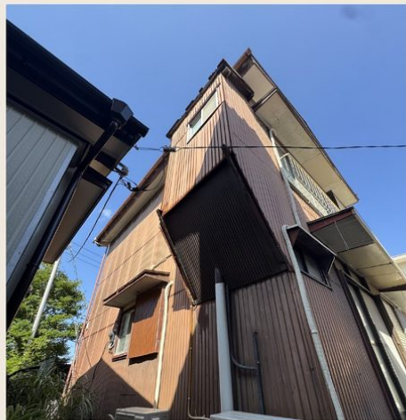
Documenting the exterior to send to the renovation company.
