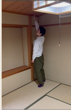
Checking the attic hatch for water damage and structural issues.
